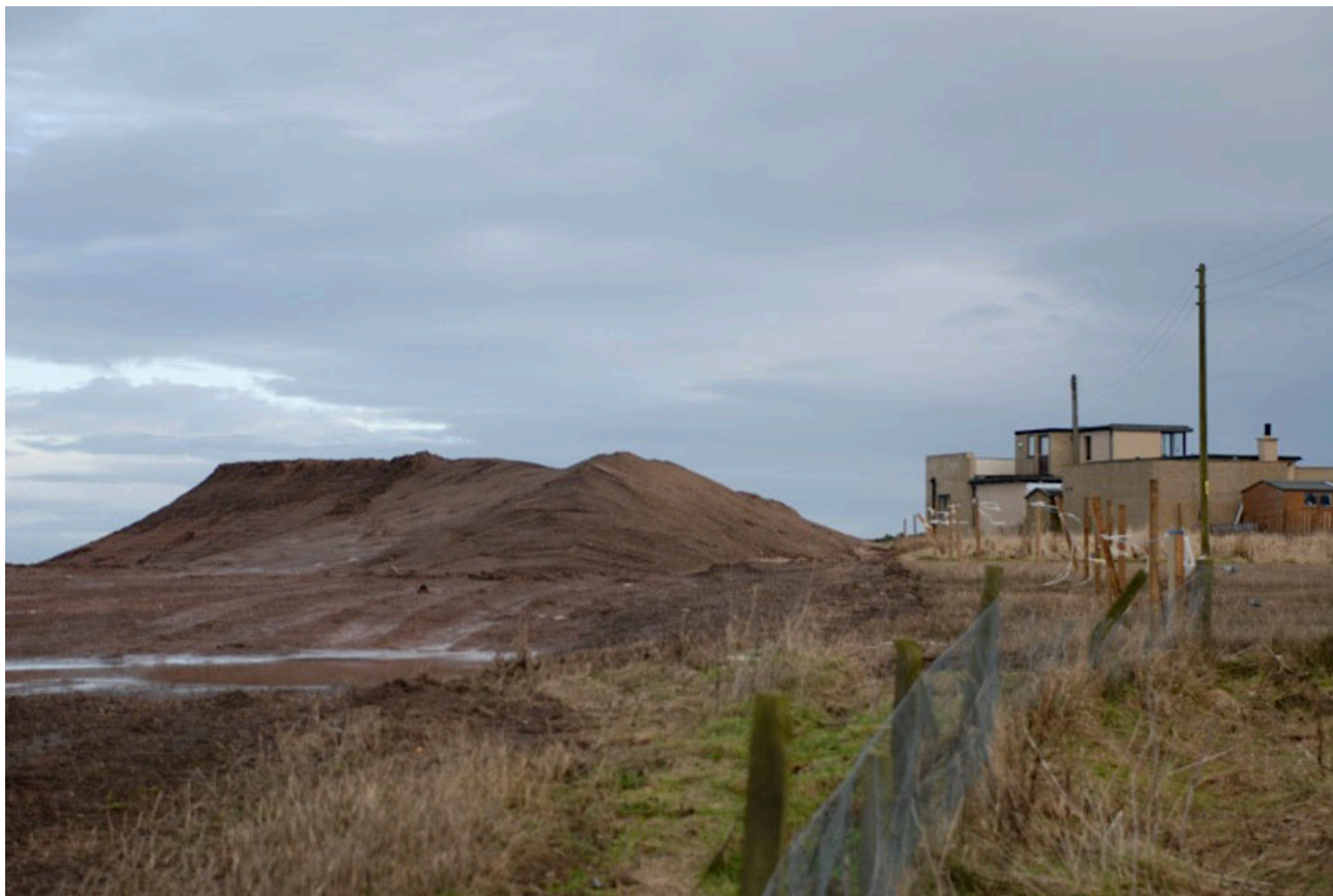
Figure 11 Bund constructed behind Hermit Point
